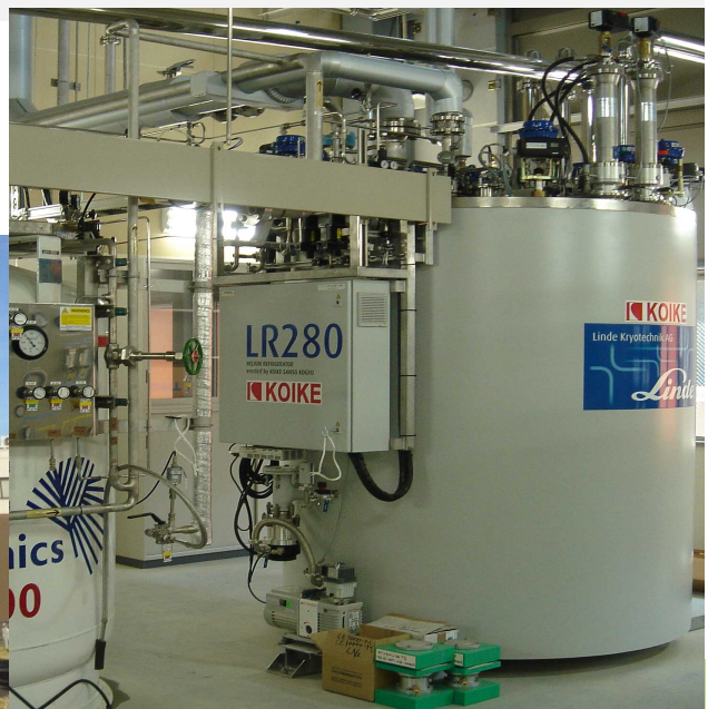
Helium liquefier/refrigerator
